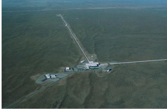
Figure 1: LIGO facility at Hanford, WA. This facility comprises of two arms stretching out 4 kms and perpendicular with each other; the arms are channels for laser beams to pass through <sup>[1]</sup>
